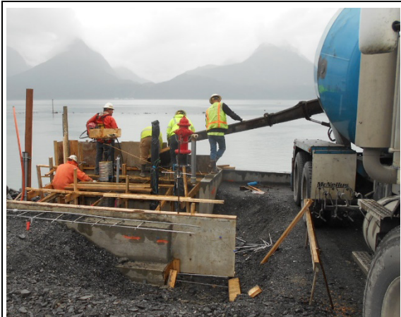
Placing concrete for utility pad retaining wall
