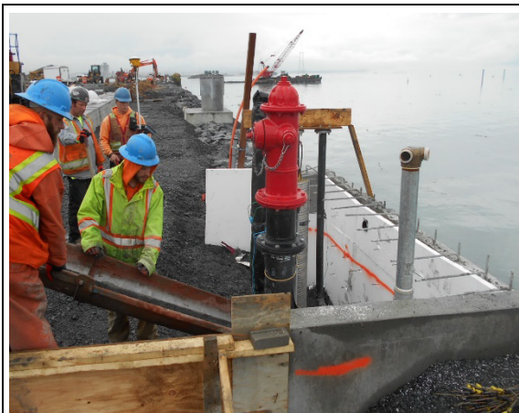
Placing slurry fill around utilities at pad area
