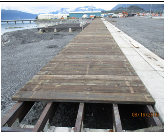
Boardwalk deck planks laid on glulam beams
