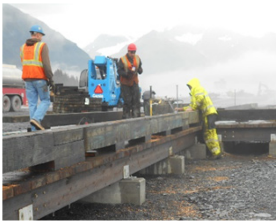
Installing bullrail on top of boardwalk deck
