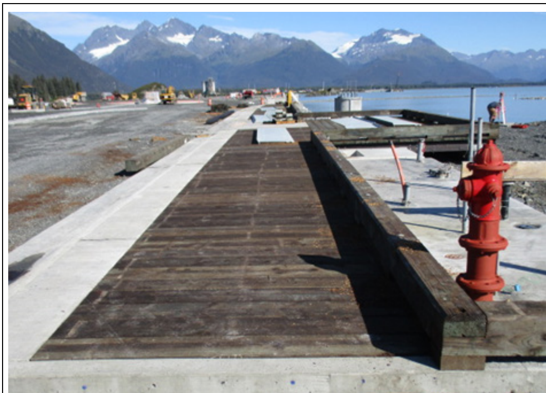
Concrete curb and sidewalk, boardwalk deck with bullrail, and concrete utility pad
