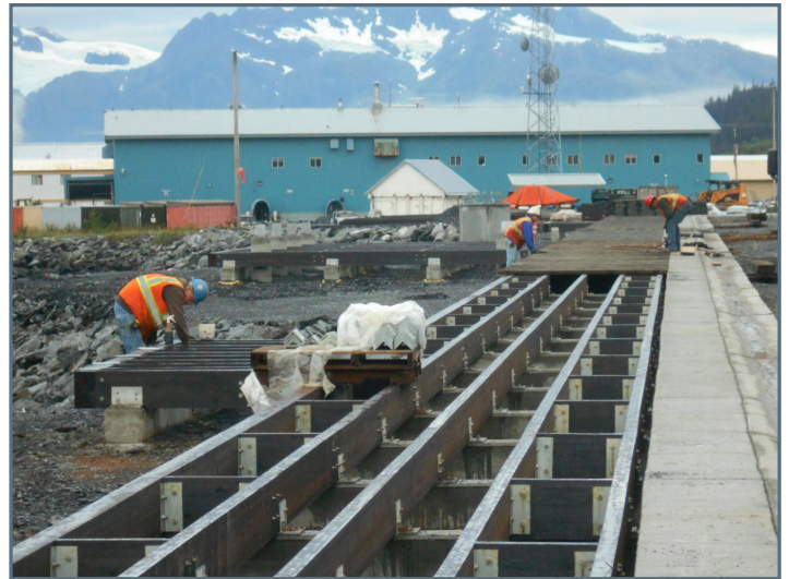
Attaching timber decking on glulam beams and solid blocking between the beams
