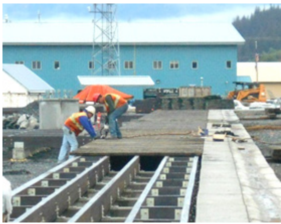
Attaching boardwalk deck planks to glulam beams
