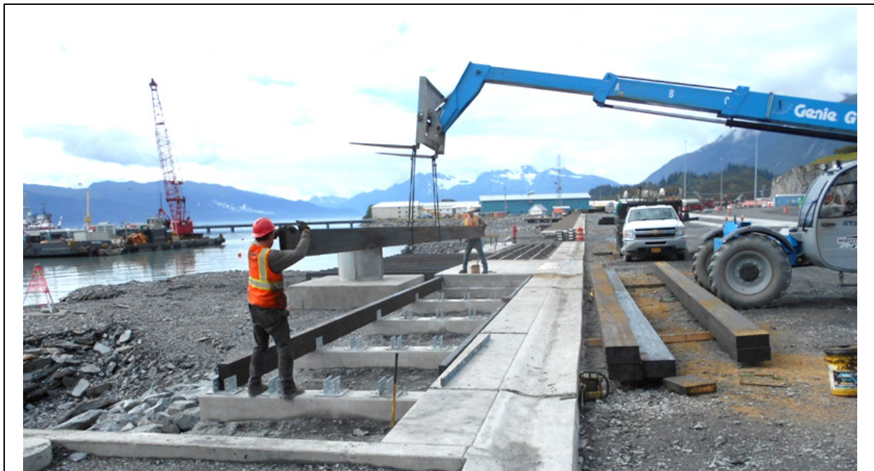
Placing 40 foot lengths of 12 inch deep glulam beams on concrete sleepers to support decking for boardwalk
