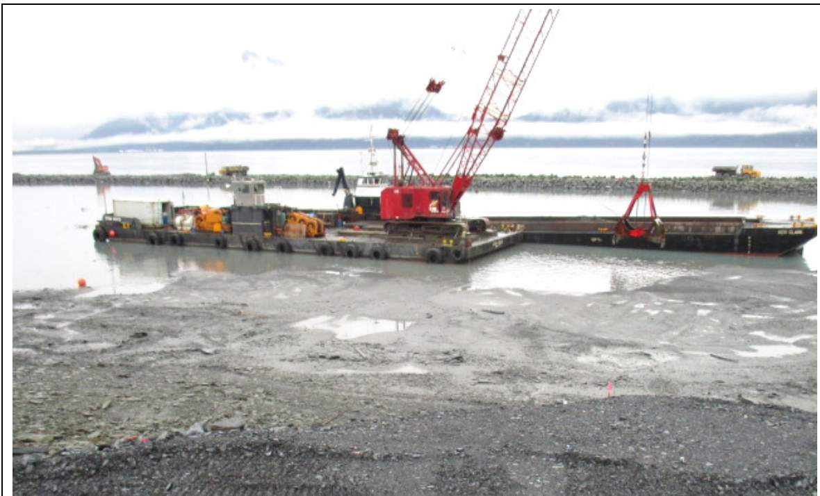
WMC dredging sediment to -14 foot depth at west portion of the mooring basin (south breakwater is beyond)
