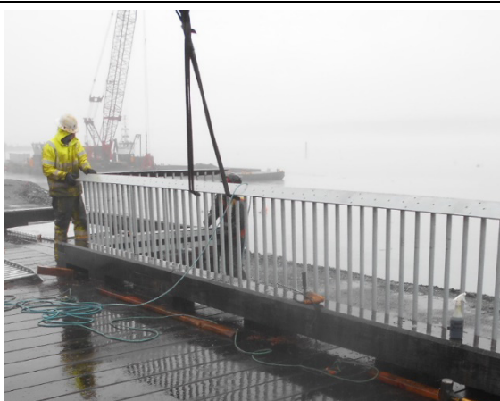
Placing section of guardrail along bullrail
