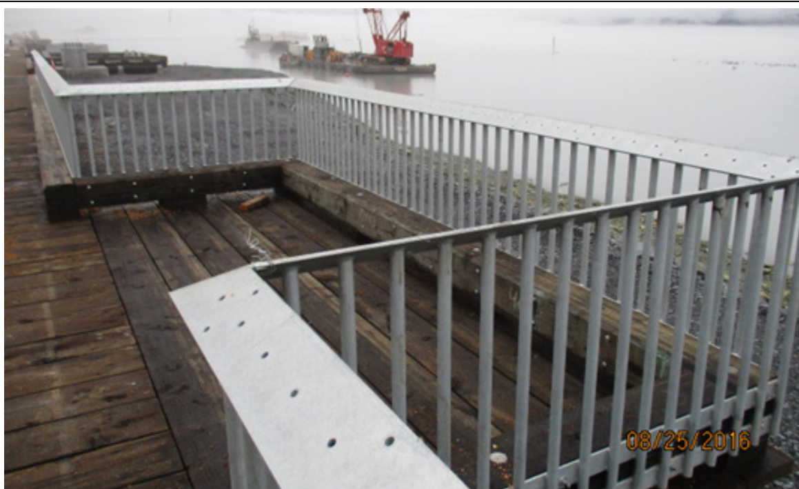
Guardrail with top plate attached to bullrail at rest area. Timber handrail will be bolted on the top plate.
