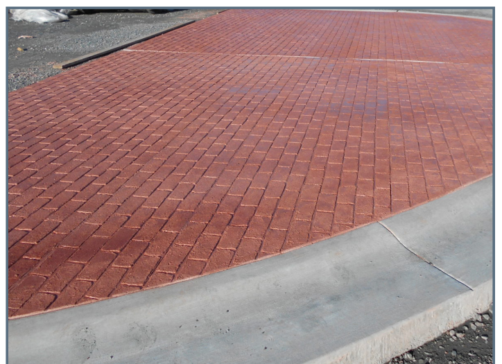
Brick pattern imprinted on red concrete that separates east access traffic from parking spaces
