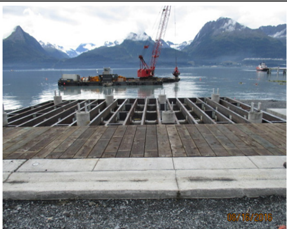
Curb, boardwalk, picnic area platform (framing)
