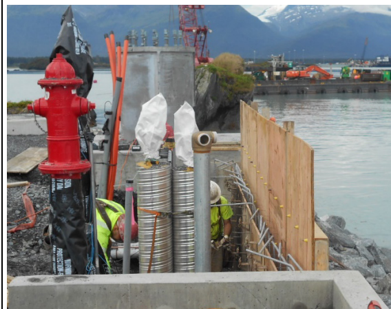
Forming retaining wall for utility pad at ramp
