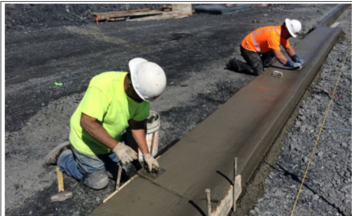
Laborers hand finish and cut contraction joints into fresh concrete curb & gutter placed by machine
