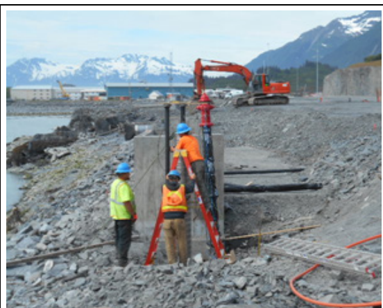
Installing fire hydrant assembly at ramp abutment
