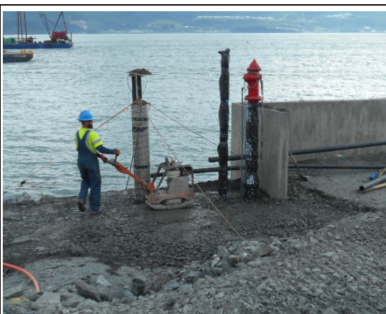
Compacting fill at water system risers and hydrant
