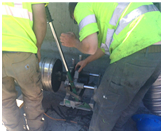
Fusing arctic pipe for backflow preventer at east ramp
