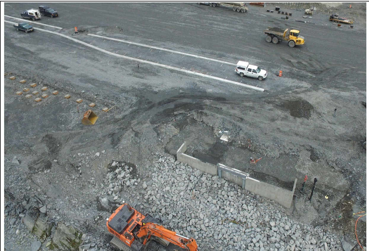
Facing north, formed sleeper keys for boardwalk (mid-left), curbs for landscape island to separate upper parking and water side drive (top left), Ramp 1 (west) abutment, fire hydrant and backflow preventer (lower right); backhoe shaping fill below abutment retaining wall (bottom). Photo by J. Talbott
