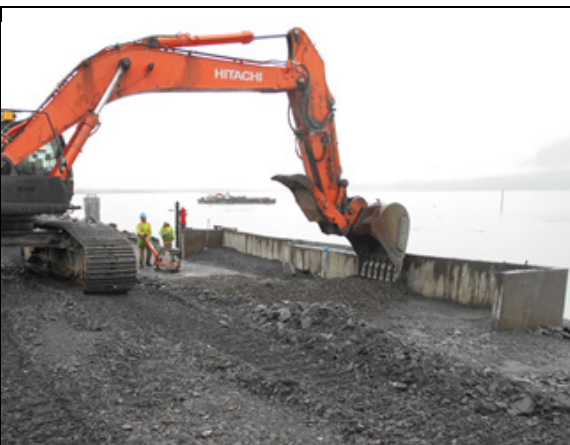
Backfilling Uplands side of retaining wall at ramp
