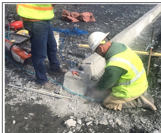
Saw cutting end of curb for clean joint
