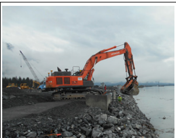
Placing riprap on slope at ramp retaining wall
