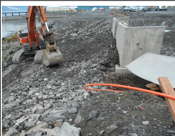
Shaping fill to place filter rock and riprap at ramp
