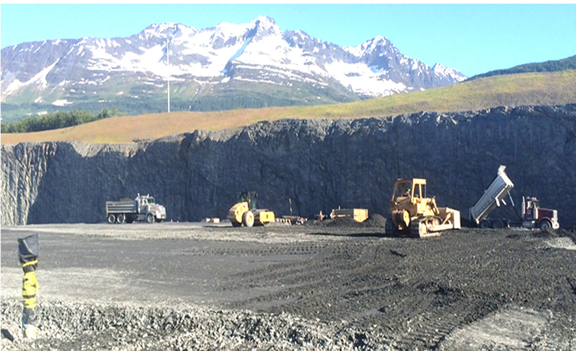
Dumping, grading and compacting crushed gravel to provide finish grade for curbs and pavement
