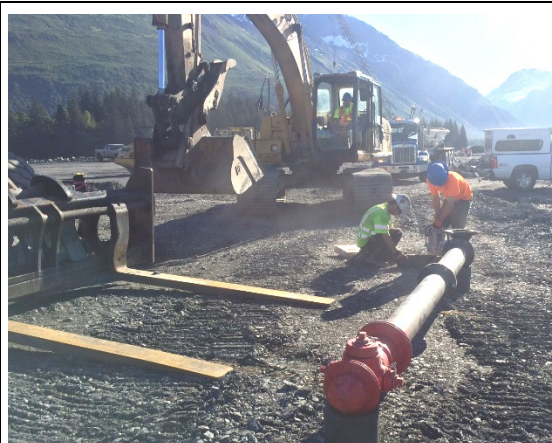
Preparing to install fire hydrant assembly
