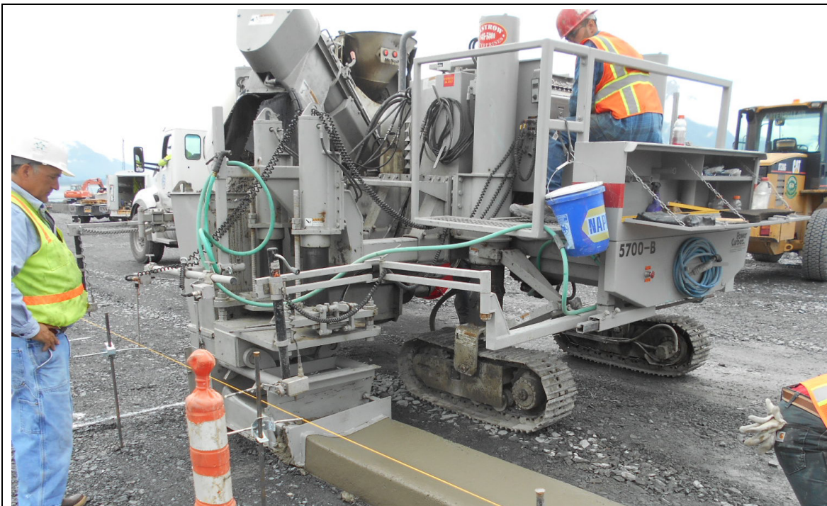
Machine follows a string line on stakes and uniformly extrudes concrete for rolled curb and gutter
