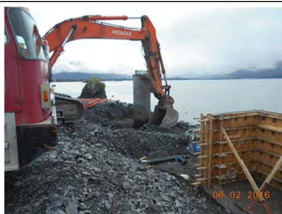
Backfilling around high mast light pole foundation
