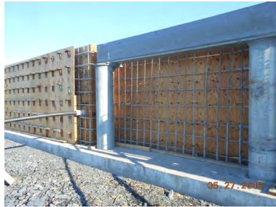
Partially formed retaining wall for ramp abutment
