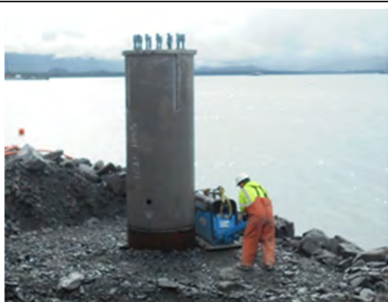
Compacting backfill at high mast light foundation
