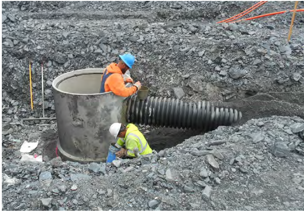
Grouting around storm drain pipe connection to manhole
