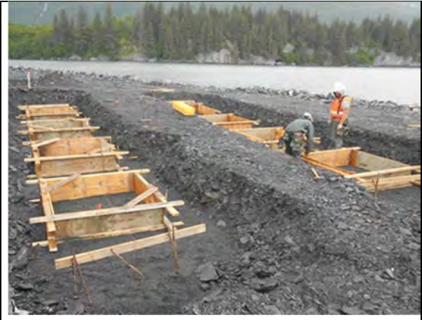
Placing forms for canopy foundations at East picnic area
