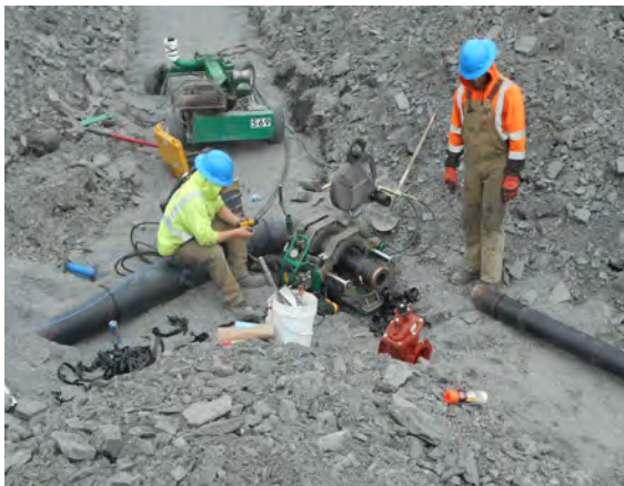
Welding HDPE reducer from water main to service line
