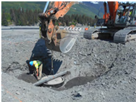
Leveling and setting base for new sewer manhole
