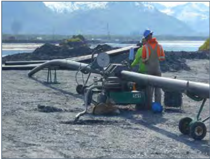
Fusion welding HDPE pipe joints
