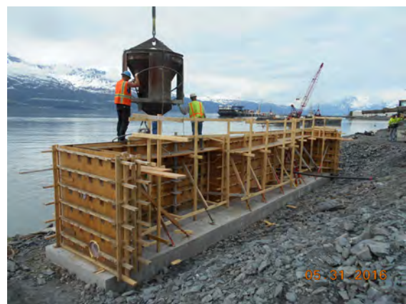
Placing concrete for retaining wall at ramp abutment
