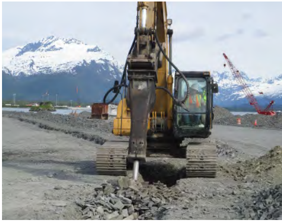
Hydraulic hammer breaking bedrock at utility trench
