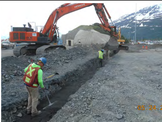
Leveling bedding before laying conduit in utility trench
