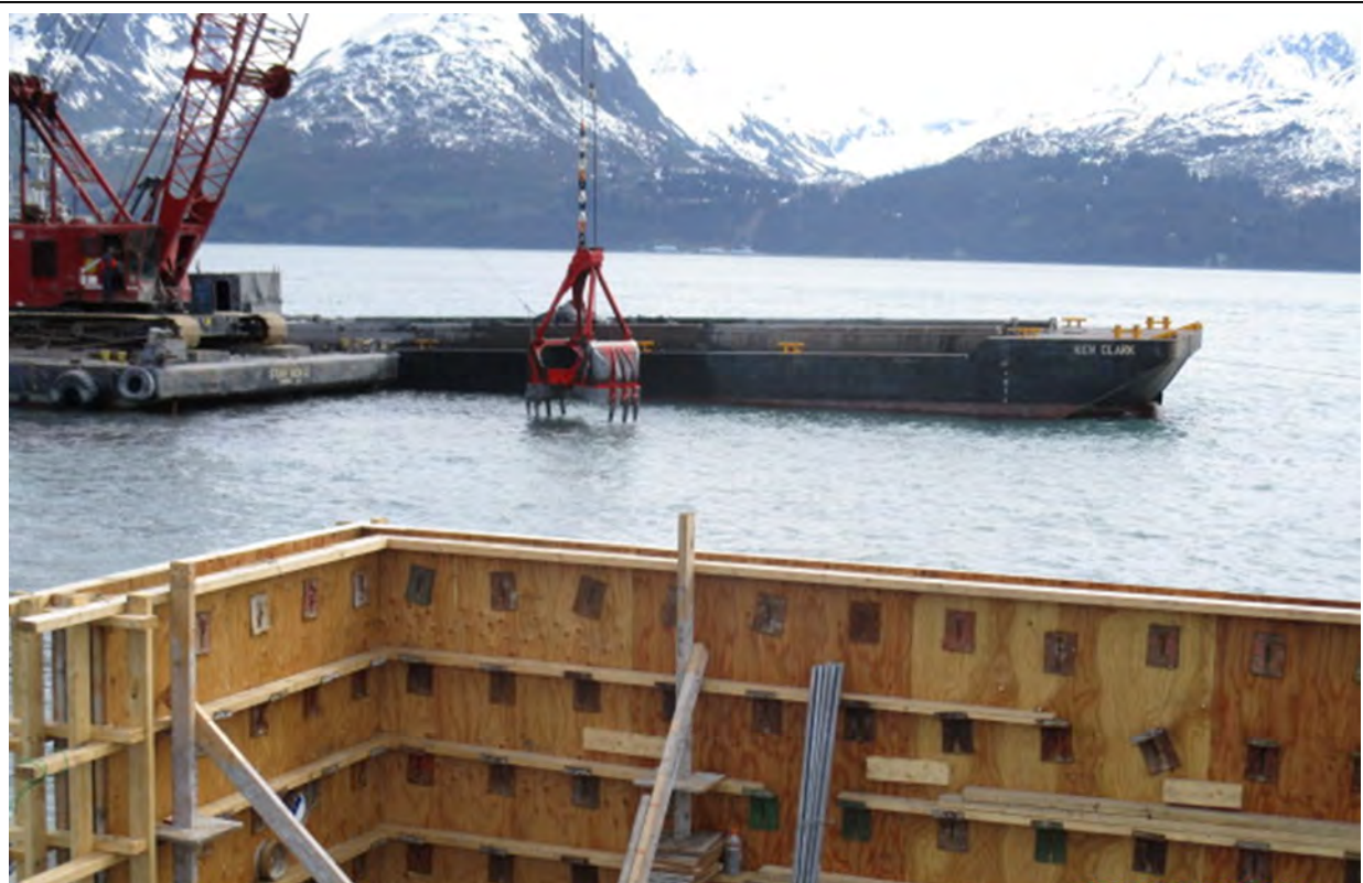
Retaining wall forms for ramp abutment (foreground) and Western Marine dredging in the float basin
