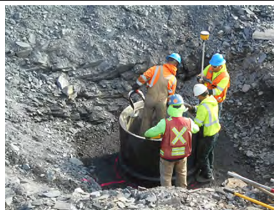
Checking elevation for storm drain manhole base section
