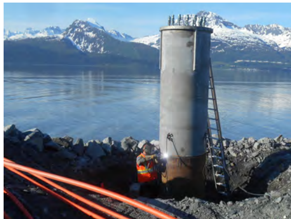
Welding base plate assembly on high mast foundation
