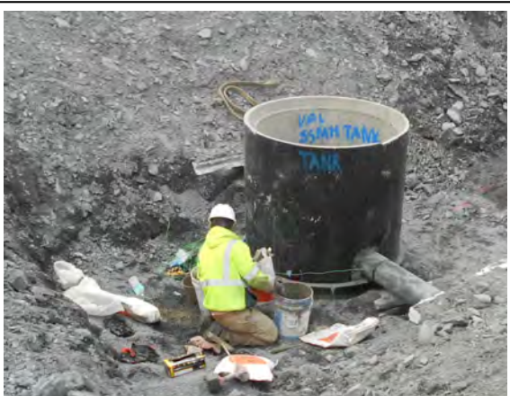
Grouting horseshoe section on sewer manhole base
