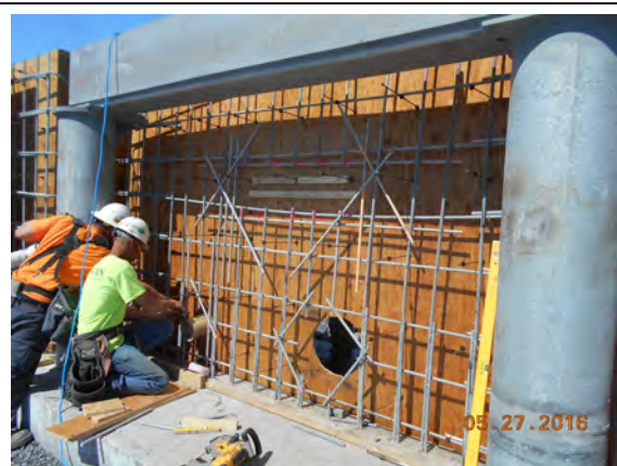
Installing utility penetration thru retaining wall rebar
