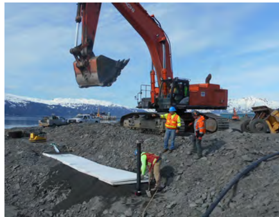
Placing rigid insulation above sewer service line
