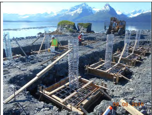
Bracing rebar spirals for foundation posts to support the canopy at East picnic area
