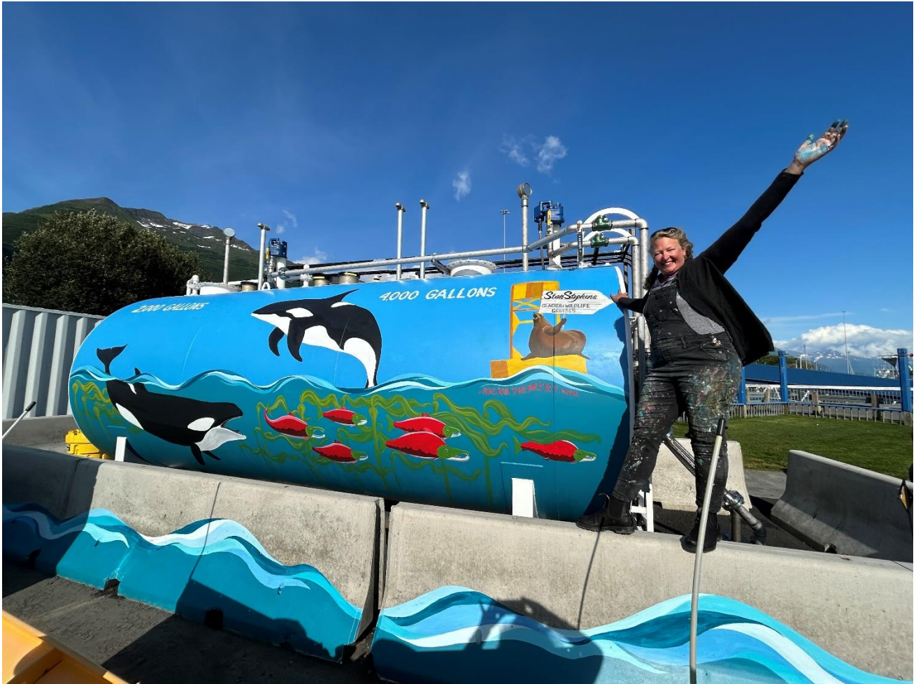
New 4K Gallon Storage Tank installed on Best Western Property
