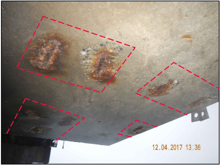
TYPICAL BOTTOM SURFACE - CORROSION SPALL
