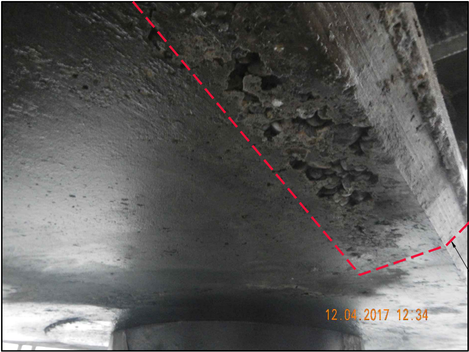
TYPICAL BOTTOM SURFACE - CONCRETE HONEYCOMB
