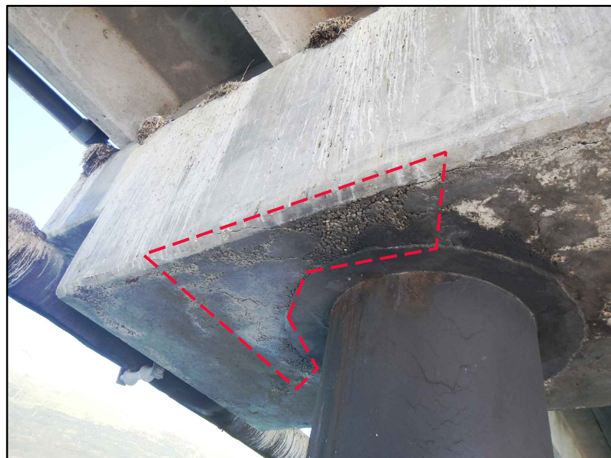
PILE CAP BENT # 23 EXISTING CONDITION NTS
