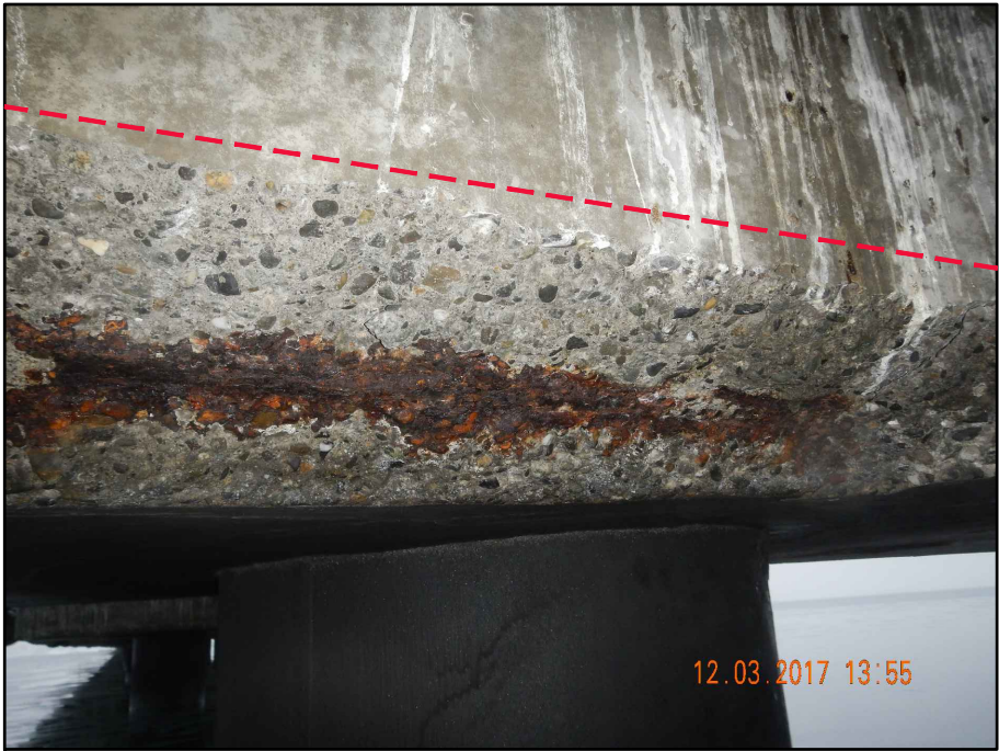
TYPICAL BOTTOM CORNER - OPEN CORROSION SPALL
