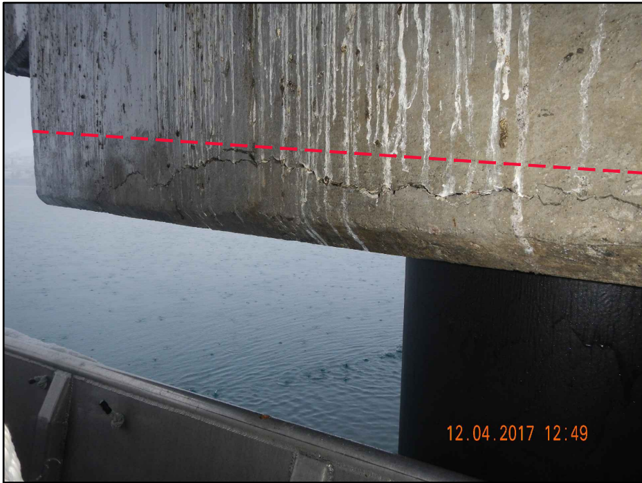
TYPICAL BOTTOM CORNER - CLOSED CORROSION SPALL
