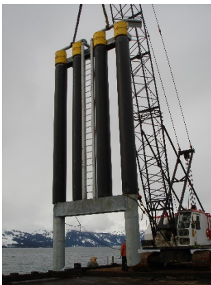
Valdez Old City Dock Fender Installation
