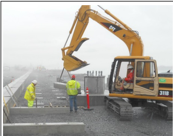
Placing precast concrete sleepers for boardwalk
