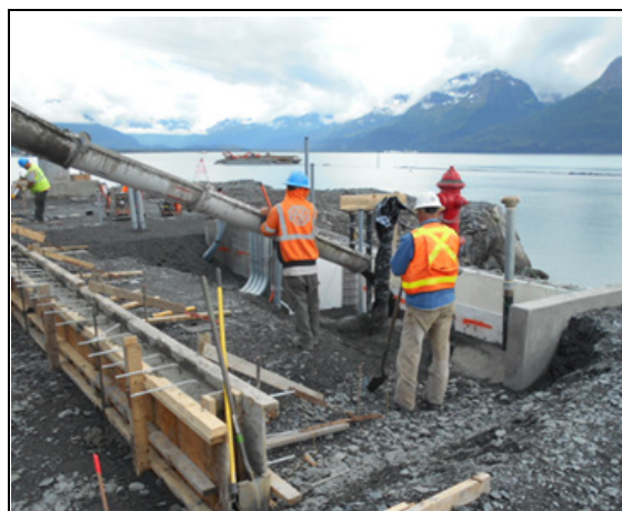
Backfilling BFP foundation with cement slurry
