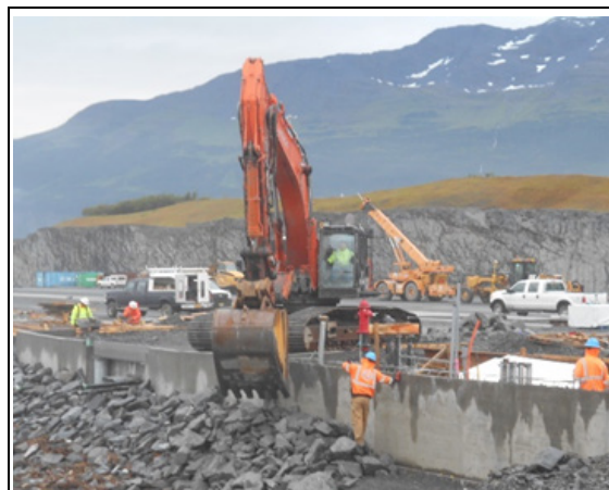
Placing riprap to protect abutment at Ramp #1
