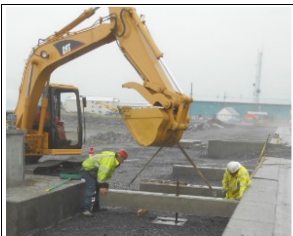
Aligning sleepers on top of concrete pads
