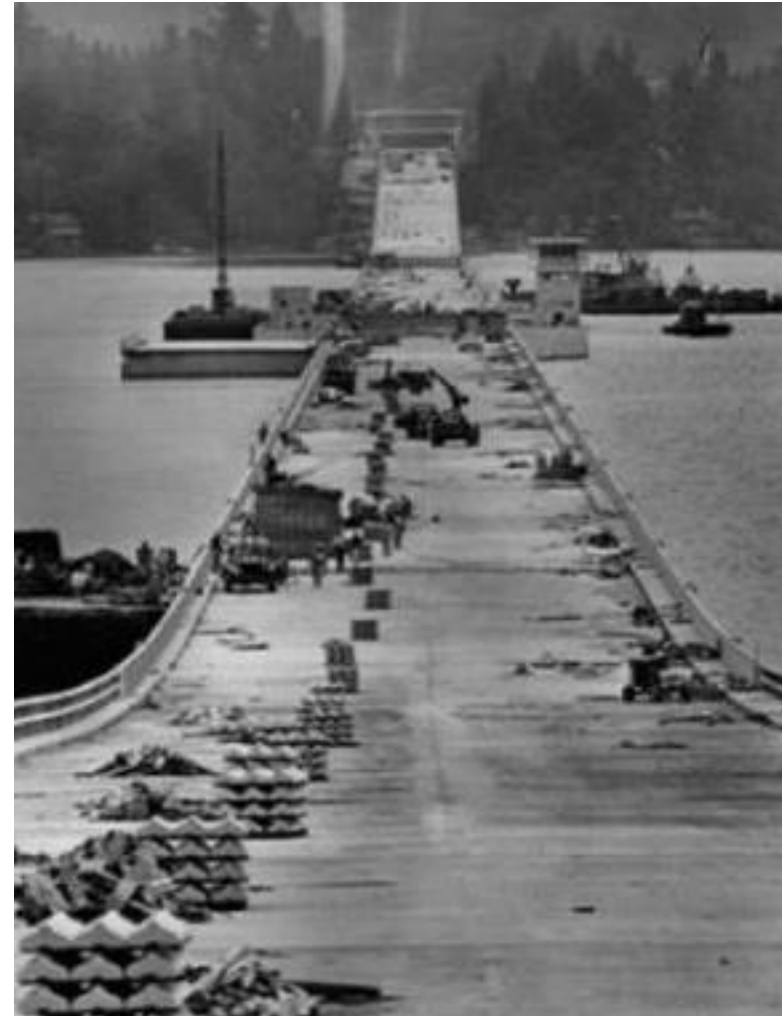
520 Bridge - Pontoons during construction
