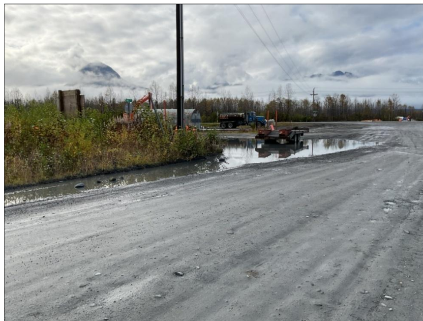
Figure 6: Lack of ditches causing standing water at N. Sawmill Dr./ Mill St. intersection
