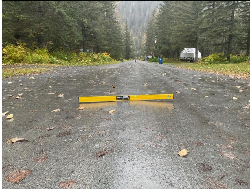
Figure 7: Defined crown on Nordic Drive
