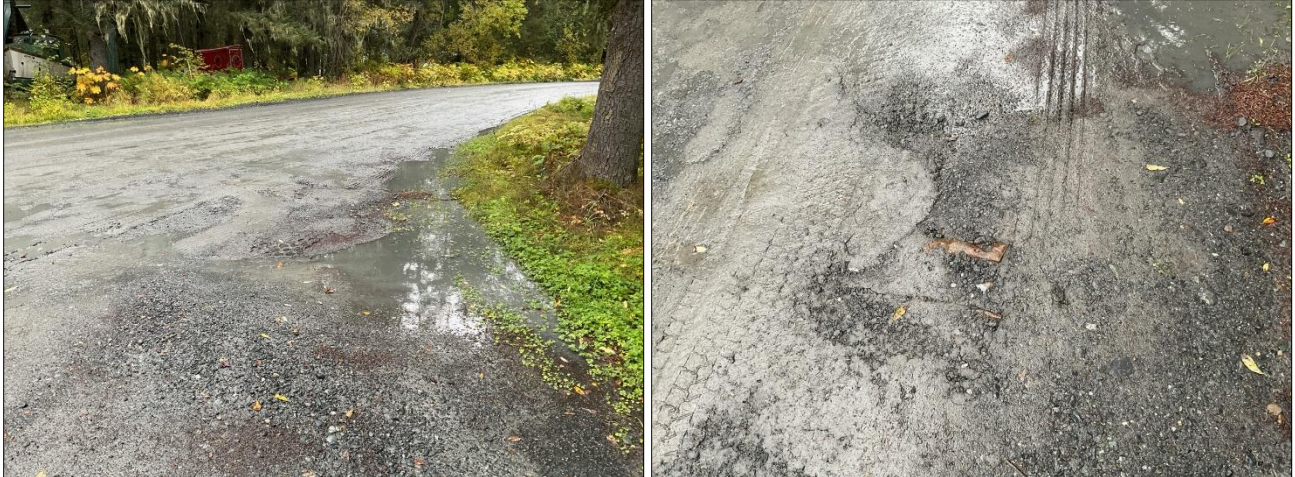
Figure 2: Intersection of Alder and Whispering Spruce - potholes and ponding above culvert (left) and remnants of crushed culvert (right)
