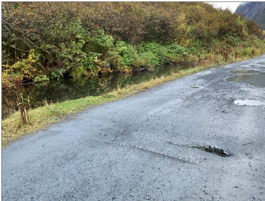
Figure 3: Damaged culvert causing standing water in ditch on Mineral Creek Road
