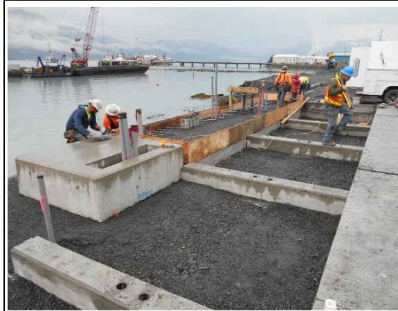
Forming utility slab and boardwalk stemwall
