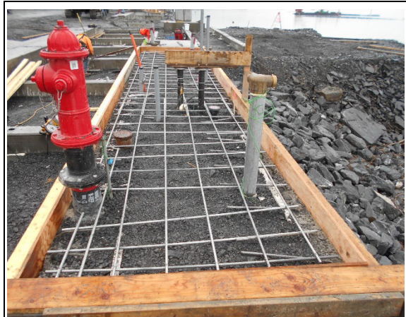
Steel mesh and forms at utility slab
