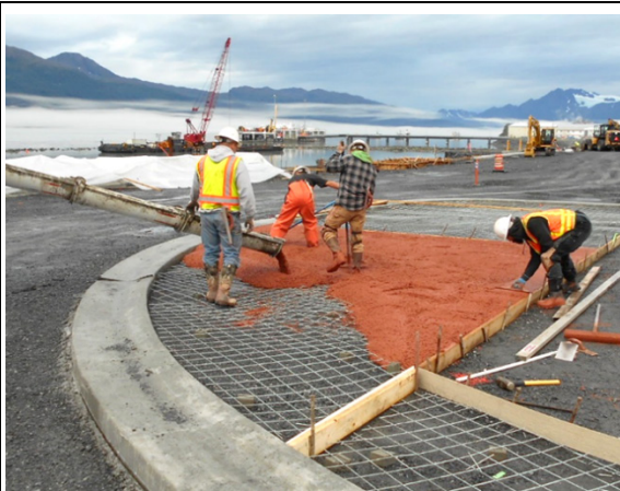
Placing red concrete for sidewalk at island area
