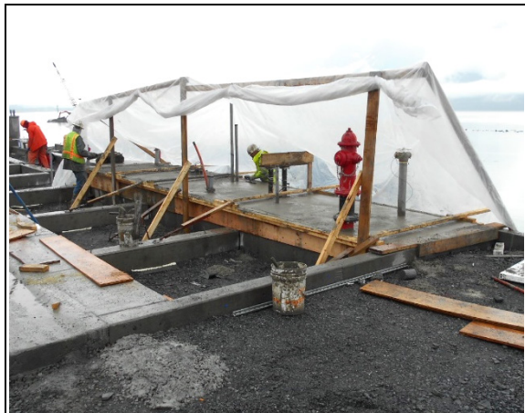
Plastic protects concrete finishing at utility slab
