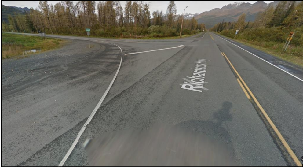
Exhibit 3. Turning from Dayville Road (East) onto Richards Highway (AK-4 North), the main route into and out of Valdez, there is limited visibility and no turn lanes to accelerate or decelerate.
