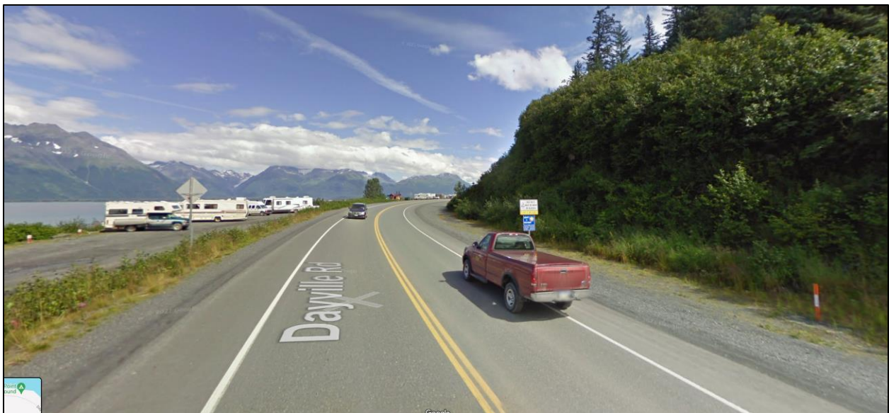
Exhibit 2. Traveling East on Dayville Road, leaving pipeline and heading towards town. Note the blind curves that are particularly challenging and dangerous when the roads are icy and snow berms further limit visibility. RVs can be seen in the designated parking area and often fill up the area in the summer; note the lack of turn lanes to allow for acceleration and deceleration. Additionally, there is no designated active transportation infrastructure, and any pedestrians or bicyclists would be sharing the road with fast-moving traffic, including the large trucks traveling to and from the refinery or pipeline.
