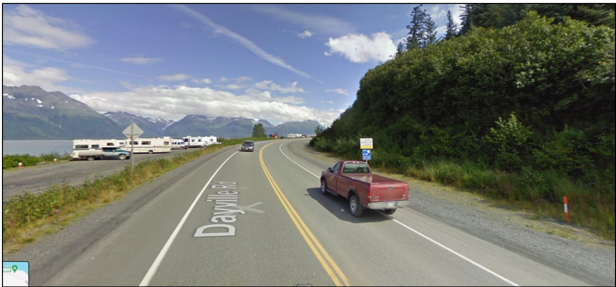
Exhibit 2. Traveling East on Dayville Road, leaving pipeline and heading towards town. Note the blind curves that are particularly challenging and dangerous when the roads are icy and snow berms further limit visibility. RVs can be seen in the designated parking area and often fill up the area in the summer; note the lack of turn lanes to allow for acceleration and deceleration. Additionally, there is no designated active transportation infrastructure, and any pedestrians or bicyclists would be sharing the road with fast-moving traffic, including the large trucks traveling to and from the refinery or pipeline.
