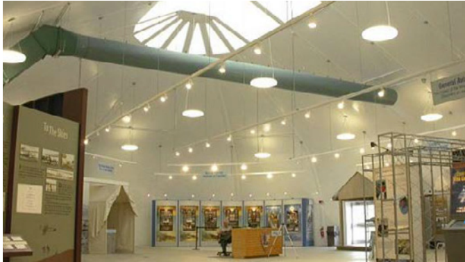
Interior of tension membrane structure
