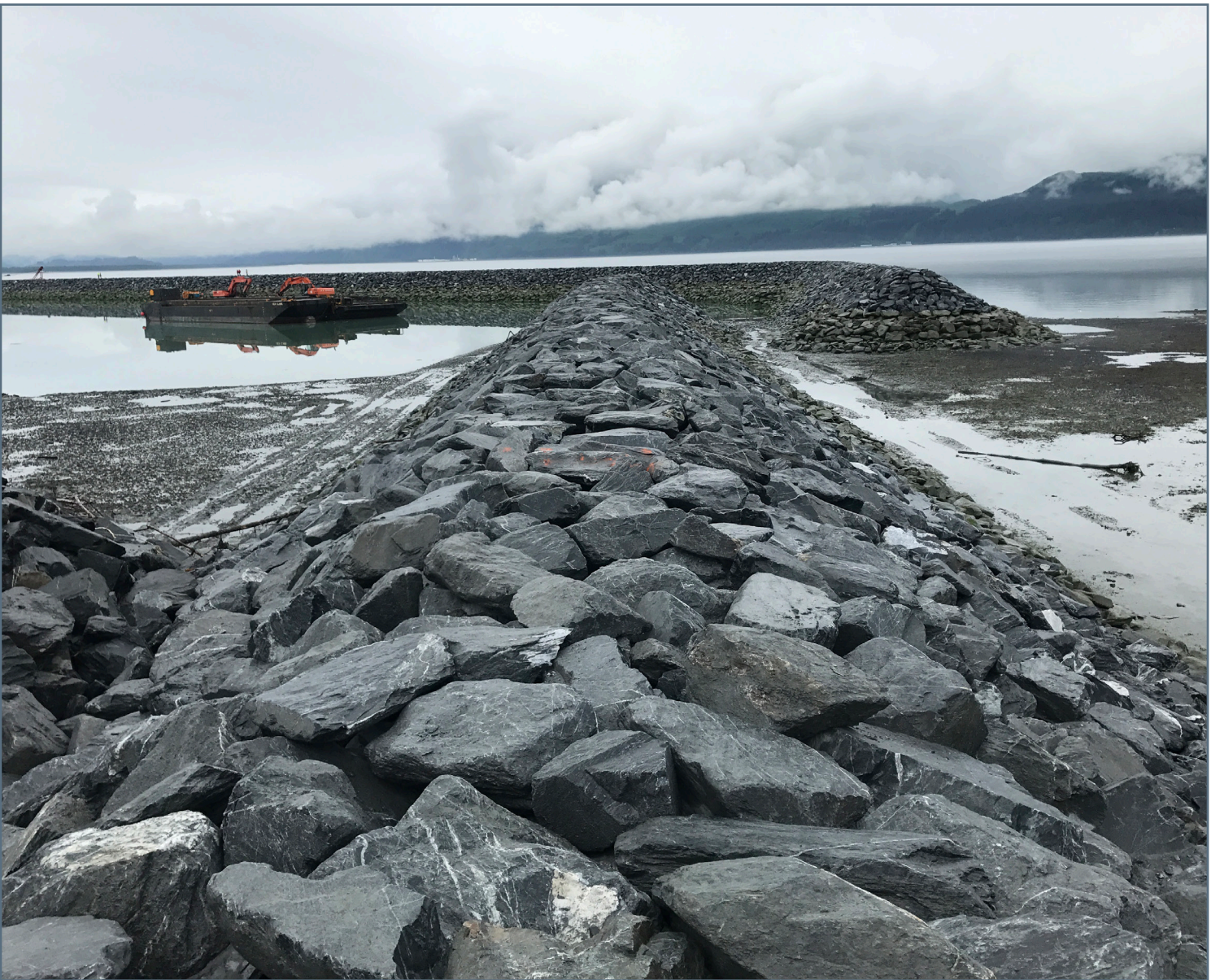
USACE – WMC Pre-Final Inspection Stub (West) Breakwater looking toward South Breakwater
