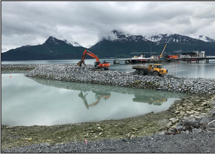
Completing Stub Breakwater
