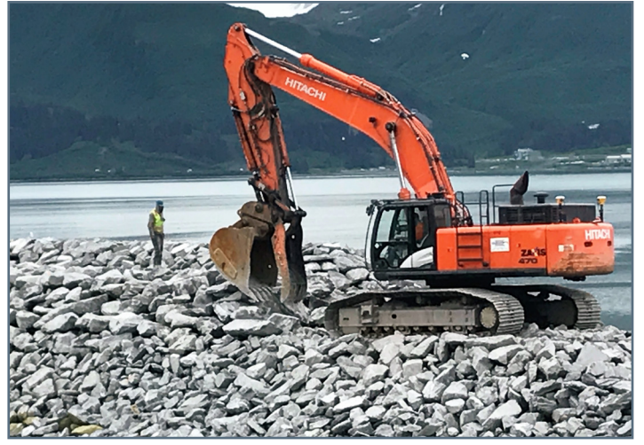
Placing armor rock on Stub Breakwater
