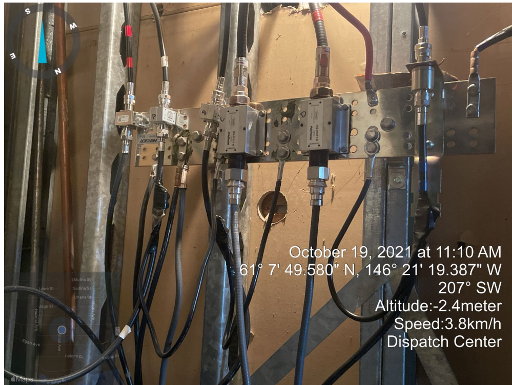
Figure 4 - Penthouse Internal Ground Bar
