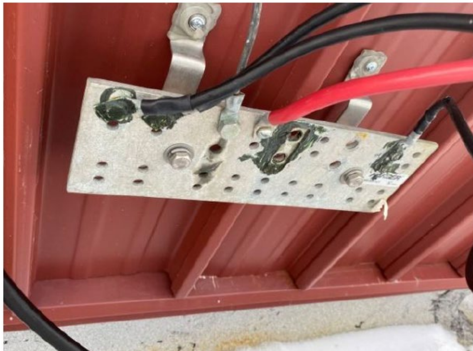
Figure 6 - Penthouse External Ground Bar
