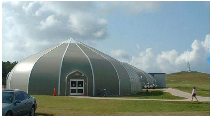
Tension membrane structure
