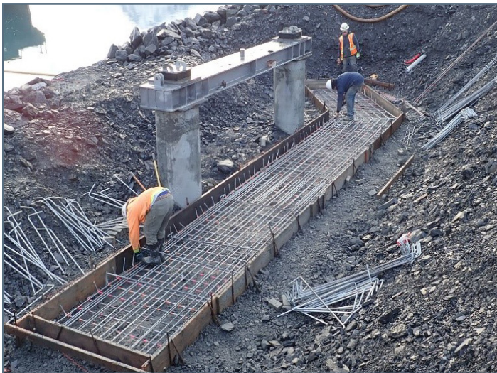
Tying rebar in footing form for bridge abutment retaining wall
