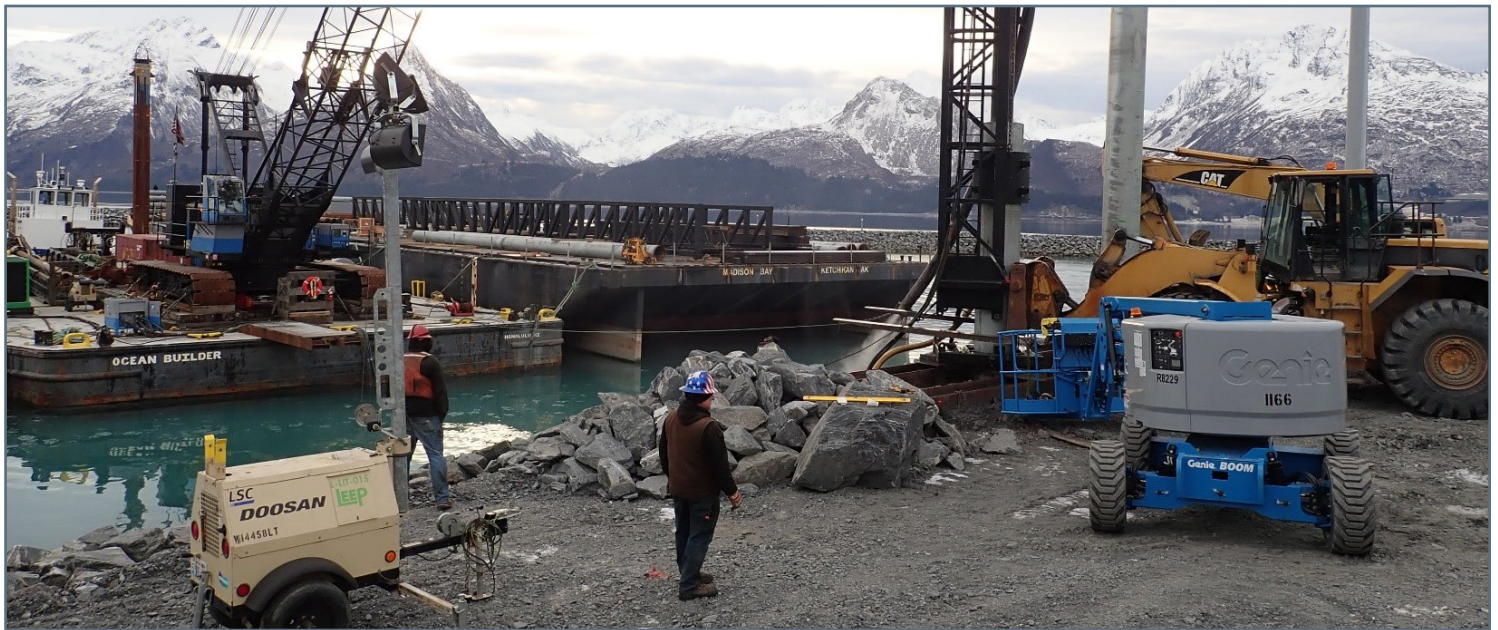
Drilling the second 30" diameter pile for DD float bridge abutment
