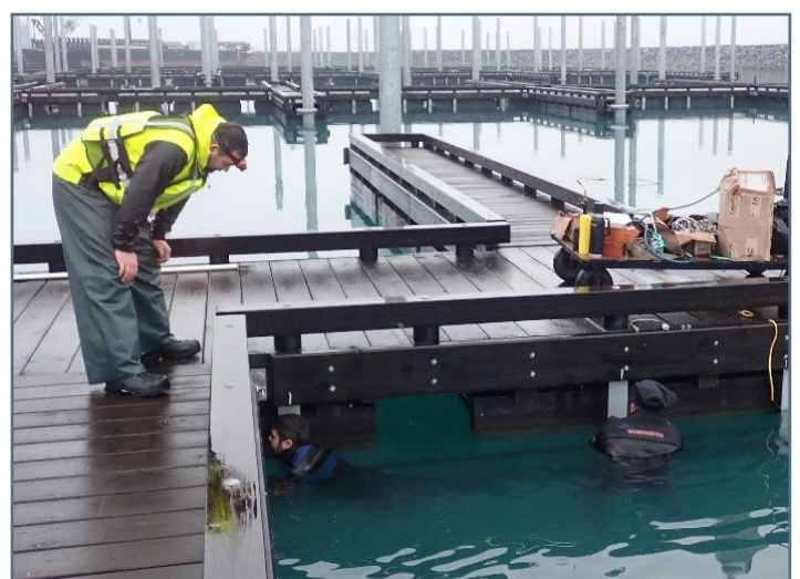
Divers attach water pipe to hangers bolted to side of floats
