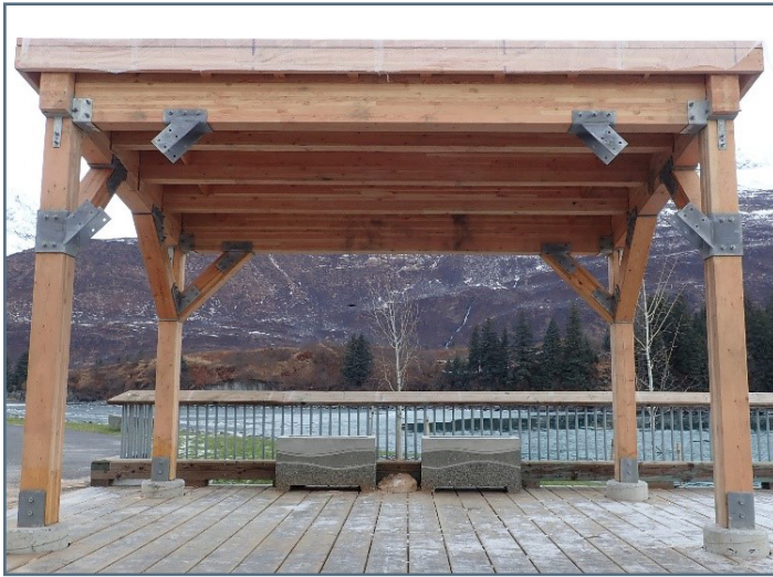
West picnic canopy almost ready for installing metal roofing
