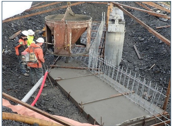
Placing concrete for footing of abutment retaining wall
