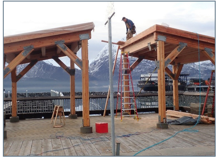
Installing tongue and groove deck on roof for west picnic canopy
