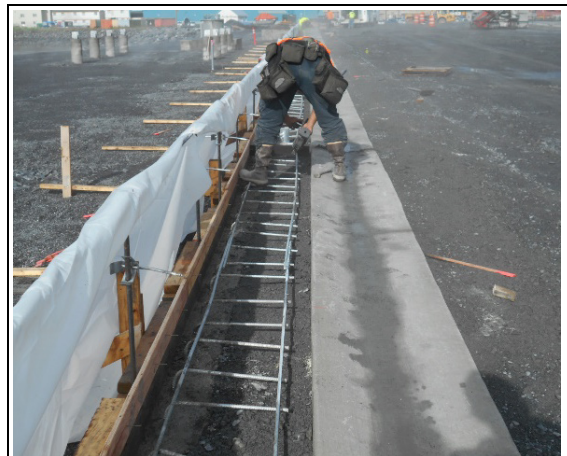
Tying rebar between boardwalk stemwall and curb
