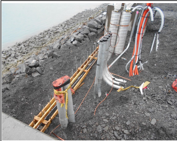
Forming footing for wall to protect utility stub-ups
