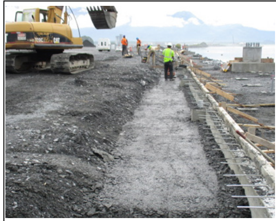
Compacting subgrade for curb along boardwalk
