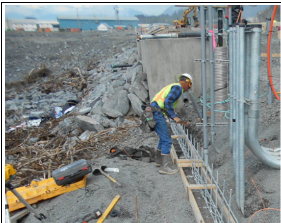
Placing footing rebar for utility pad wall
