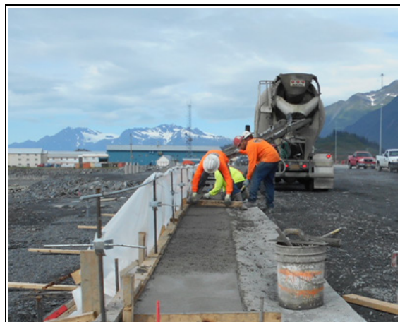
Finishing fresh concrete between stemwall and curb
