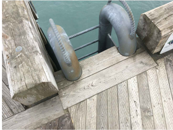
PHOTO #10 - TYPICAL LADDER TRANSITION
