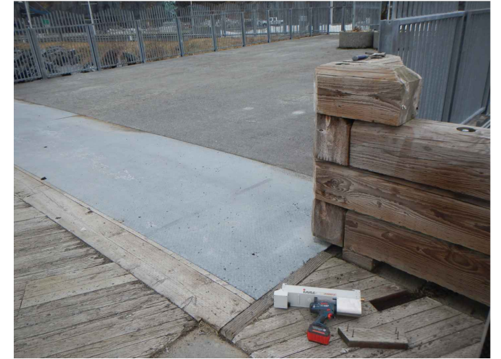
PHOTO #13 - CENTER APPROACH TRANSITION
