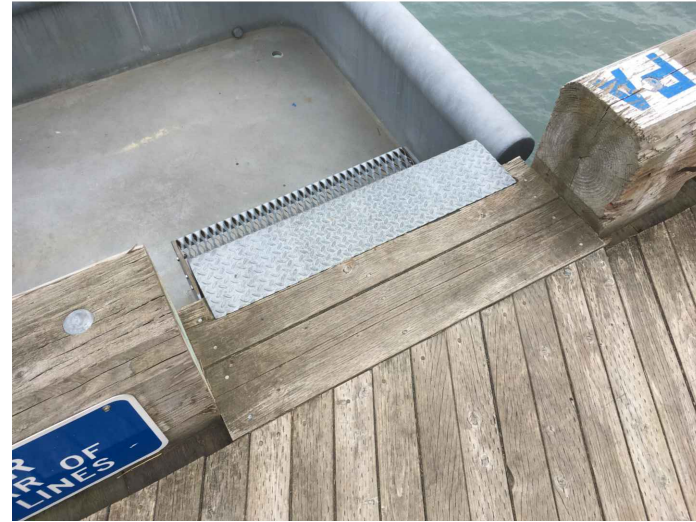
PHOTO #11 - TYPICAL FENDER STEP TRANSITION
