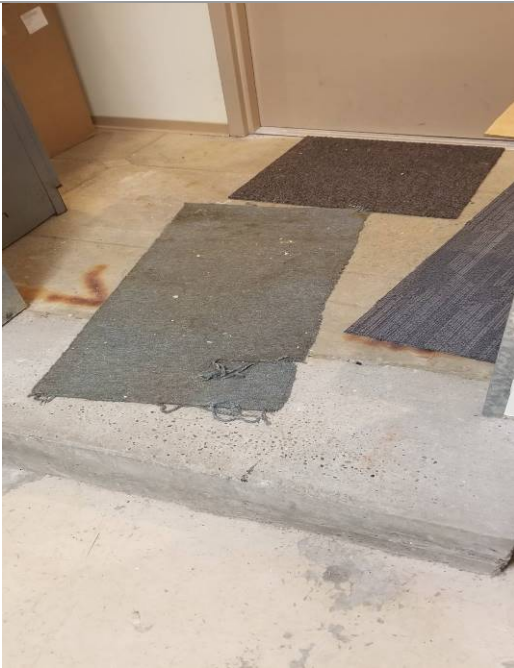
07-12219A: Rec Center; Highlight the step on both sides with safety tape or fluorescent paint to minimize potential for tripping hazard and injury.
