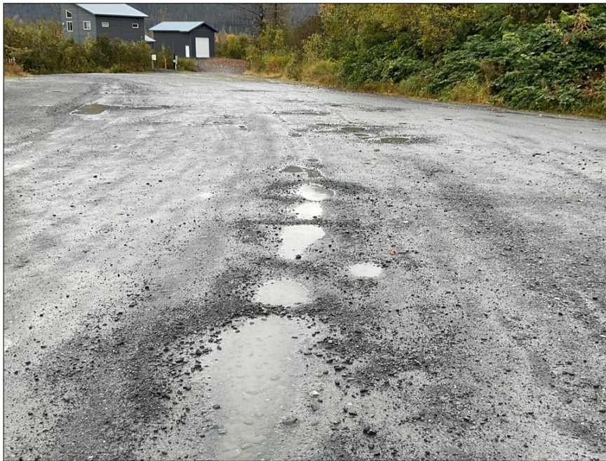
Figure 8: Potholes developing within the crown area on Cummings Way
