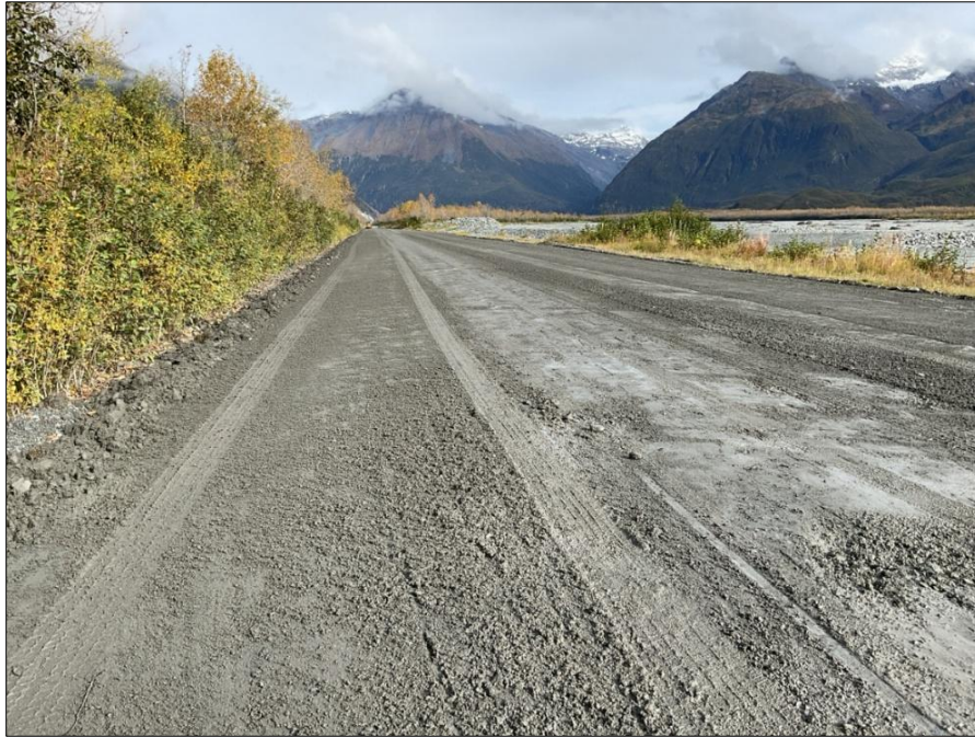
Figure 1: Berms on left created during routine grading on Glacier Haul Road
