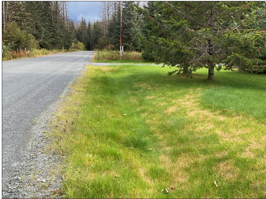
Figure 4: Well-maintained ditch on Childs Street
