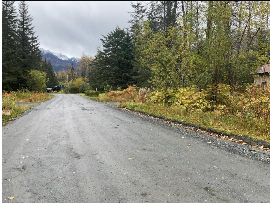
Figure 9: Surface course graded off road into berm on Chalet Drive
