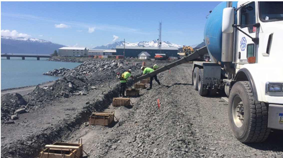
Subcontractor (Zastrow) crew placing concrete in forms for boardwalk sleeper keys
