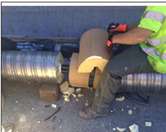
Placing insulation around fused joint in arctic pipe
