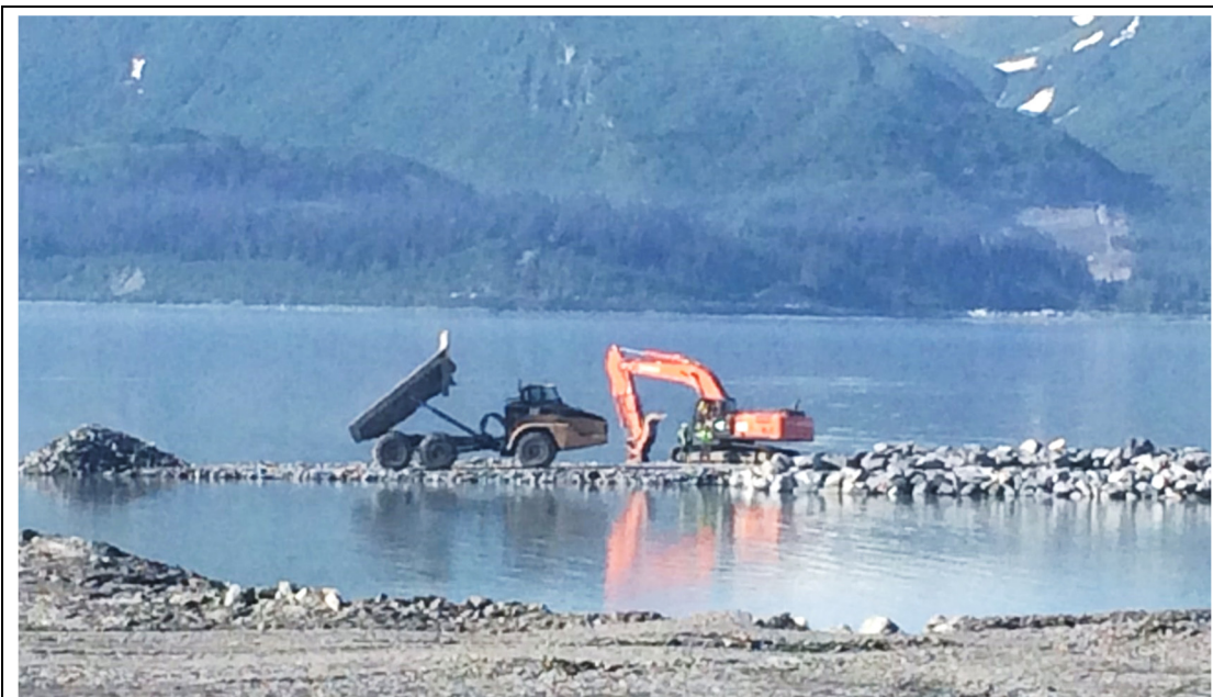
Western Marine placing rock to construct the south breakwater. Photo by J. Talbott
