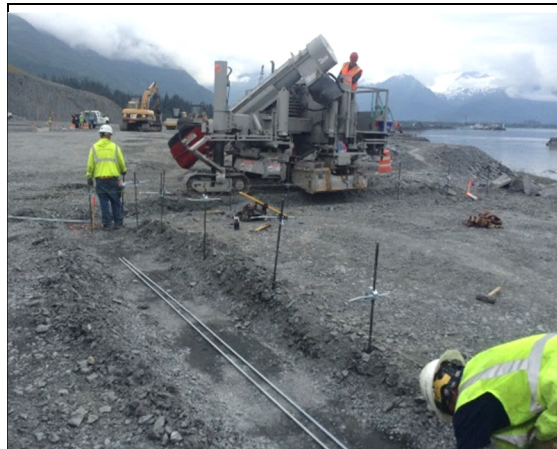
Preparing to place curb at future Wash Down Pad
