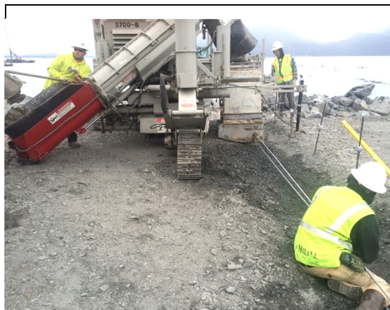
Placing steel reinforcement for curb
