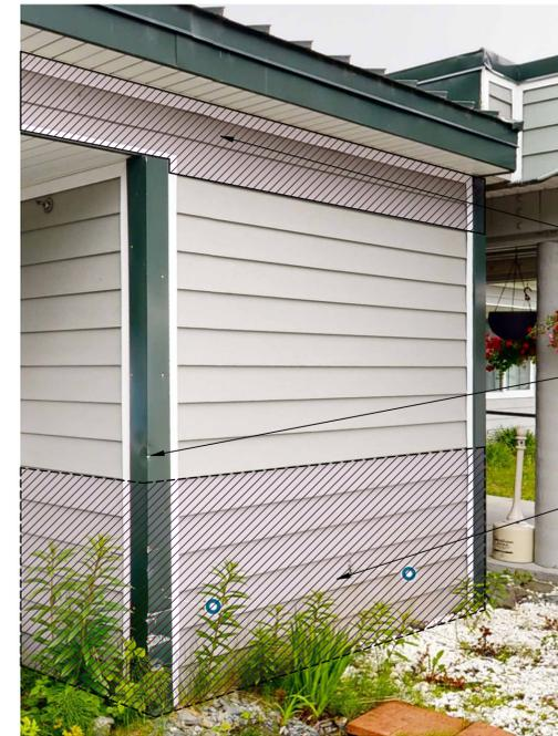
REMOVE AREAS OF BUCKLED SIDING AND TRIM; REPLACE WITH RELOCATED SIDING AND NEW TRIMS.
