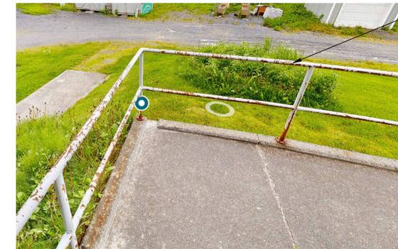
REMOVE, REFINISH, REINSTALL CORRODED HANDRAIL--ALT 1
