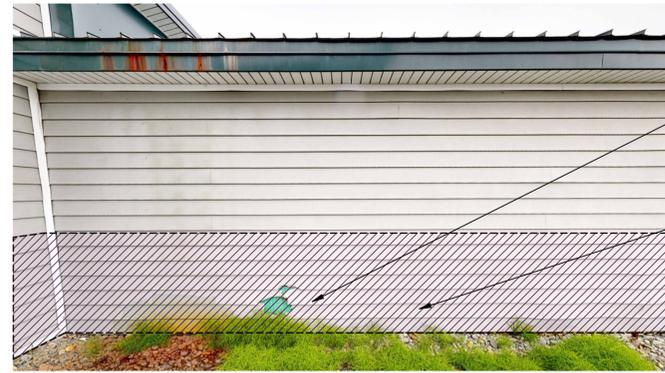
REMOVE DAMAGED SIDING; EXAMINE AND REPAIR SUBSTRATE AND WEATHER BARRIER AS NEEDED.
