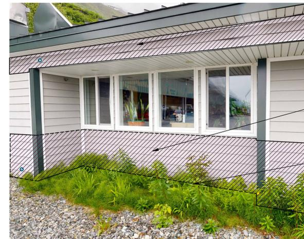
REMOVE AREAS OF BUCKLED SIDING AND TRIM; REPLACE WITH RELOCATED SIDING AND NEW TRIMS.
