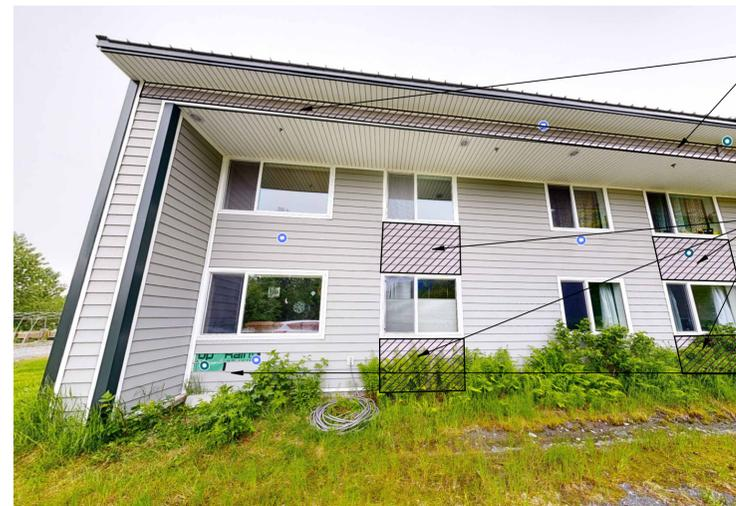
REMOVE & REPLACE BUCKLED SIDING AND TRIM; INSTALL NEW EXPANSION JOINT.
