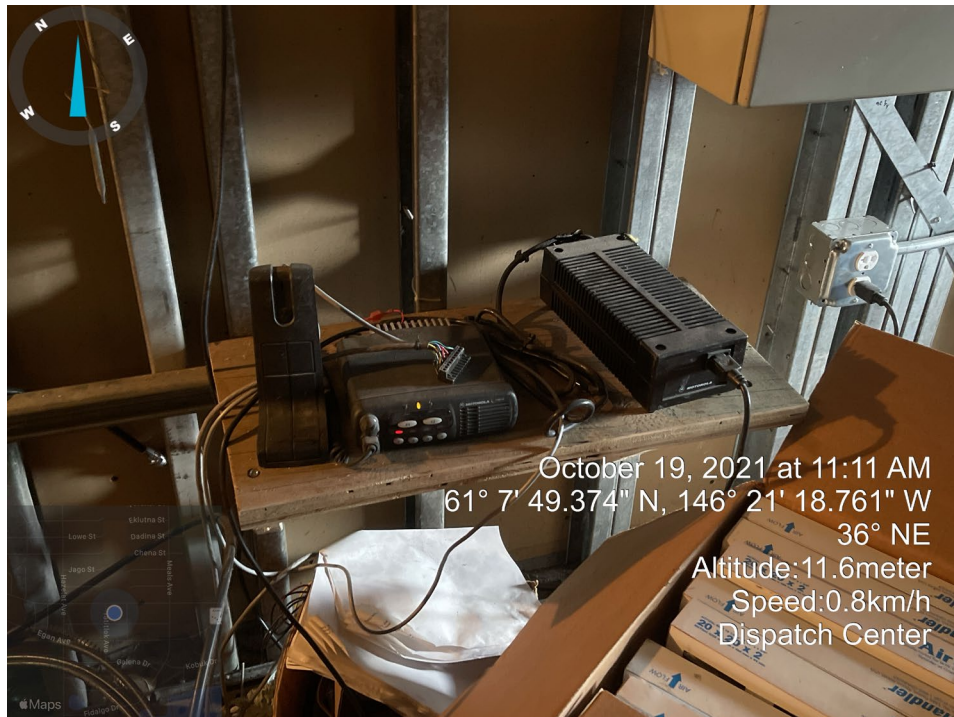
Figure 5 - Tsunami Warning UHF Radio
