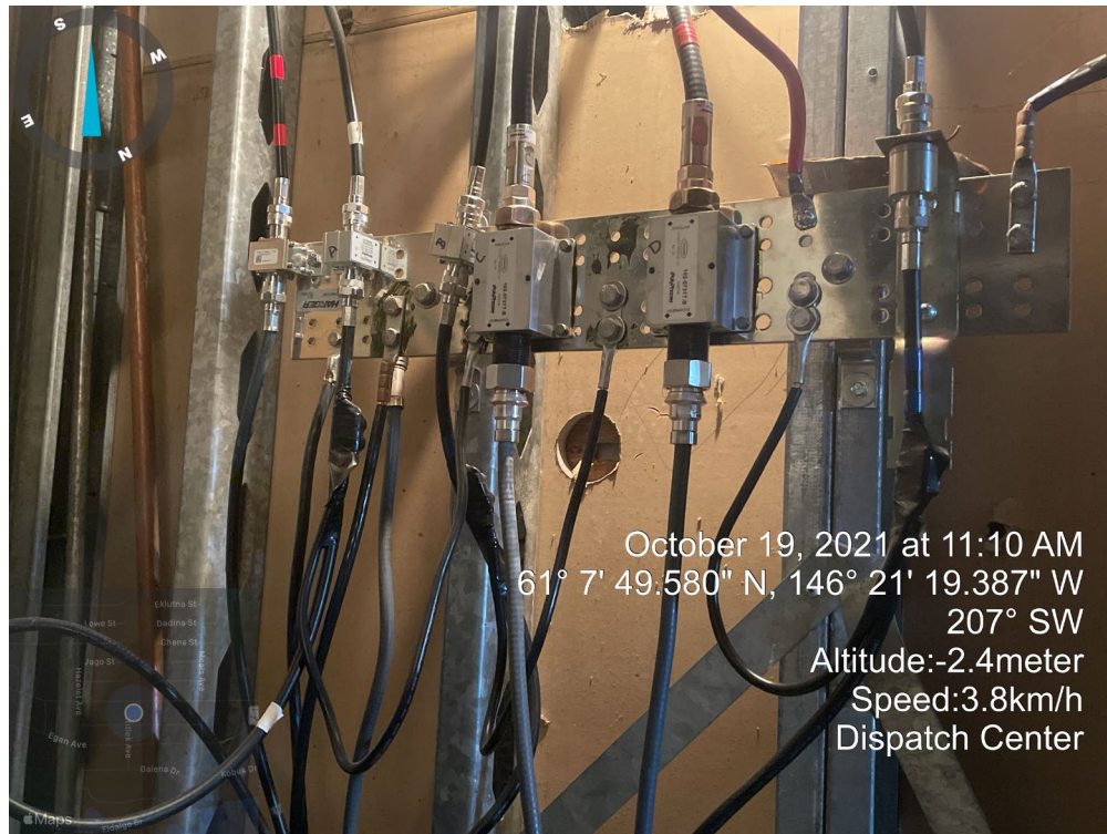
Figure 4 - Penthouse Internal Ground Bar
