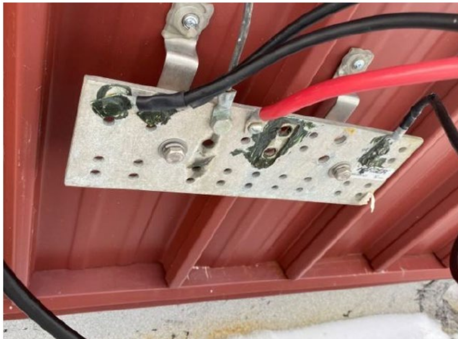
Figure 6 - Penthouse External Ground Bar
