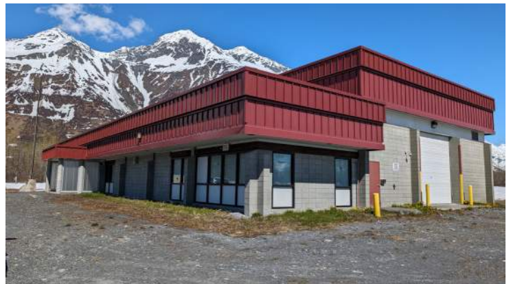
Armory Exterior Overall
