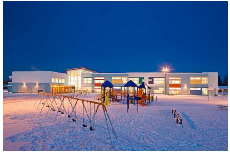
Childcare Facility - Exterior Playground
