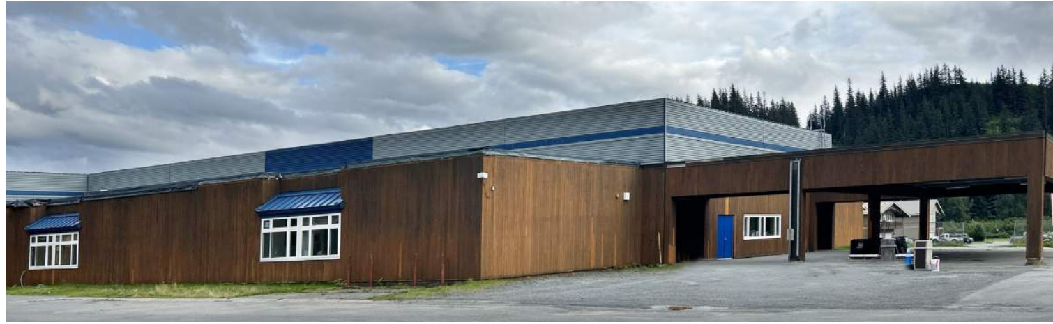
Existing covered area at west end of Hermon Hutchens Elementary
